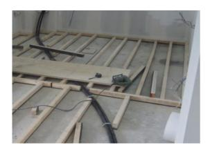
Profloor resilient batten is a composite acoustic batten which has been designed to improve the acoustic performance of concrete floors. It comprises of a close cell resilient layer adhered to a planed softwood batten.
